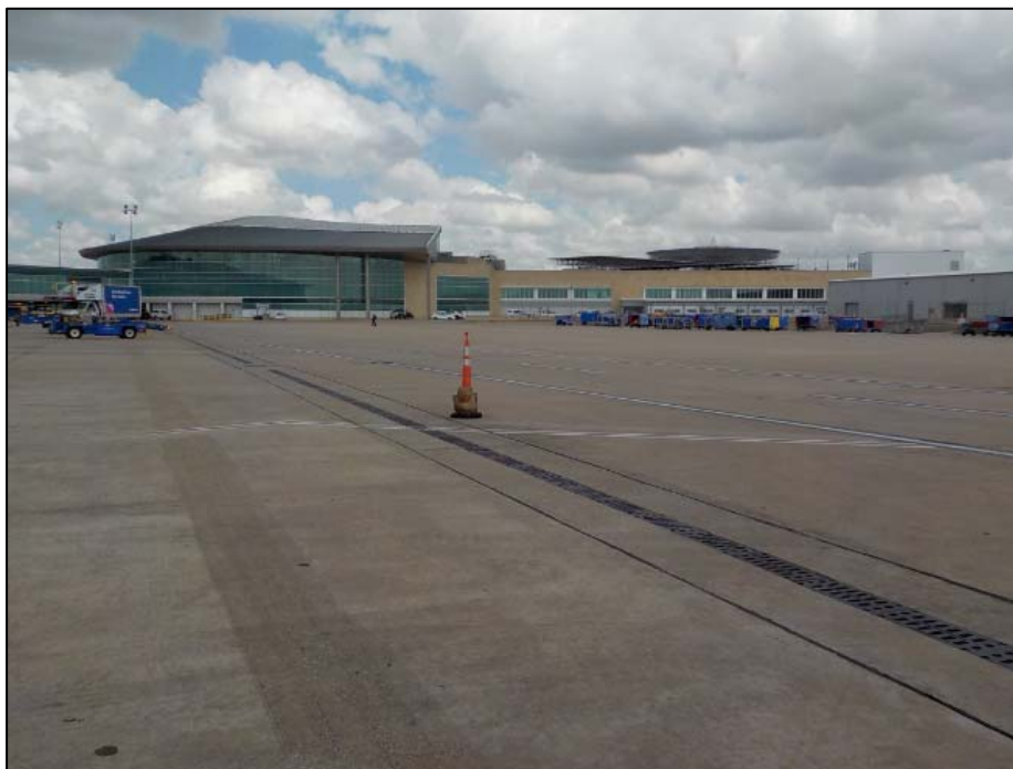
Photo 3. Overview of the eastern side of the HOU Central Terminal Building, facing west.
