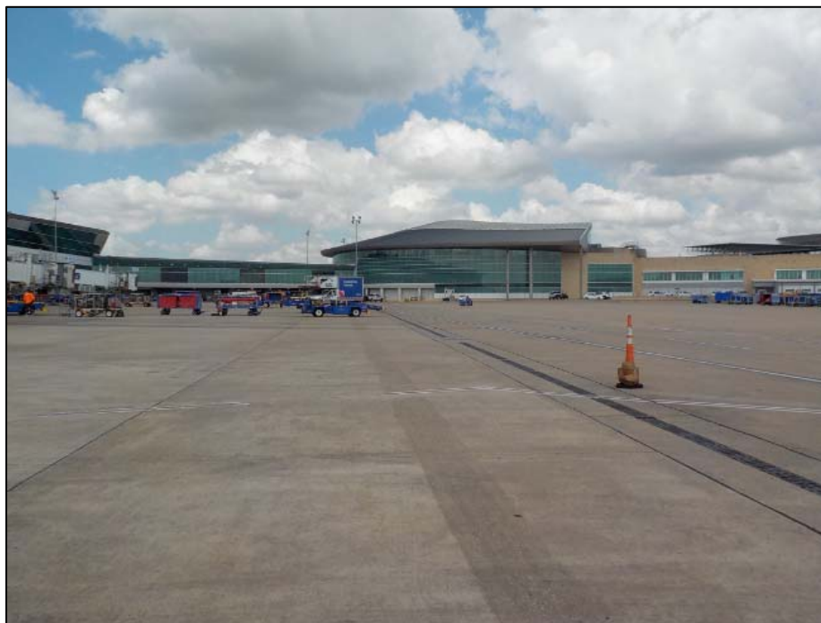
Photo 5. Another view of the eastern side of the HOU Main Terminal Building, facing west.
