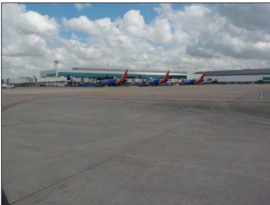
Photo 12. Overview of the West Concourse Terminal building, facing northeast.
