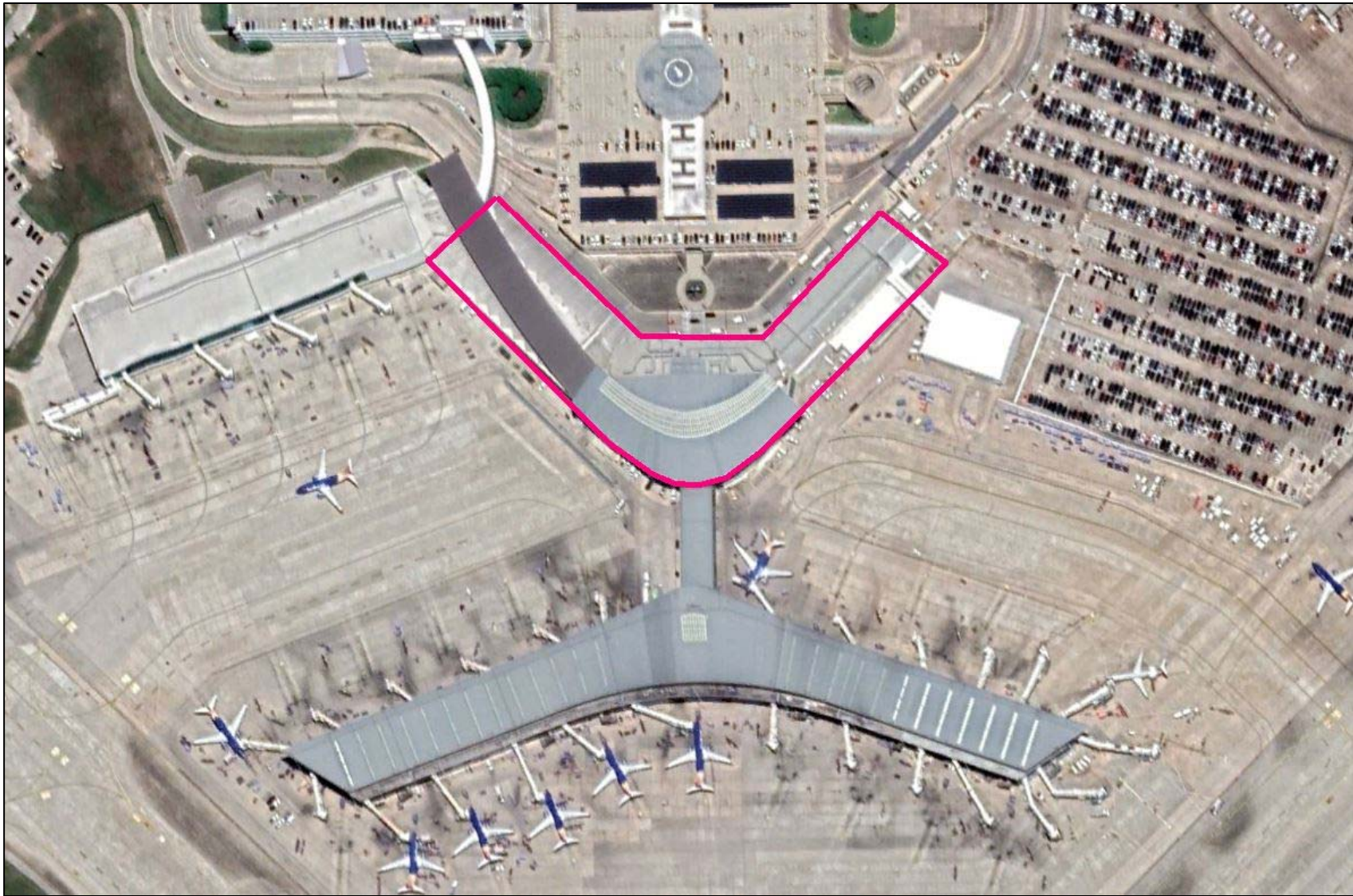
AERIAL OVERVIEW OF CENTRAL TERMINAL BUILDING
