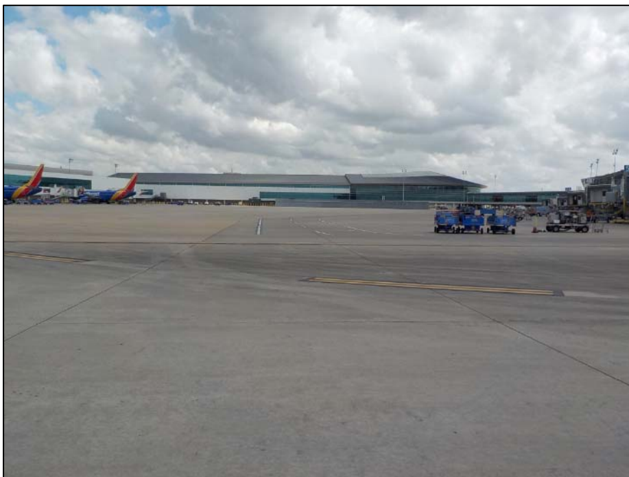
Photo 11. Another overview of the western side of the HOU Main Terminal Building, facing east.
