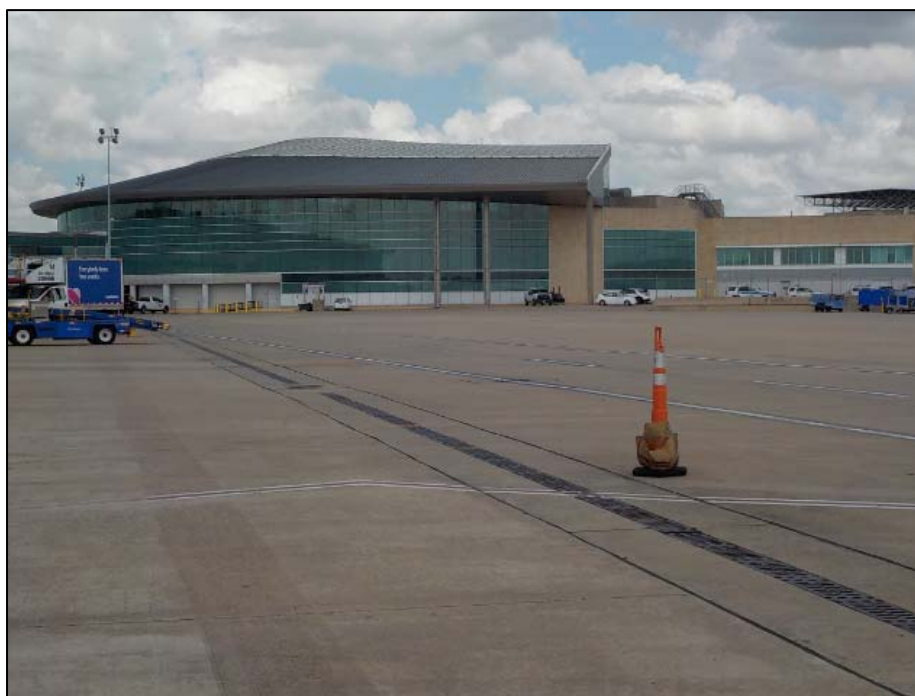
Photo 4. Another view of the eastern side of the HOU Central Terminal Building, facing west.
