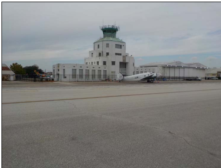
Photo 7. View of the 1940 Air Terminal Museum at the southwestern end of the project limits, facing southwest.
