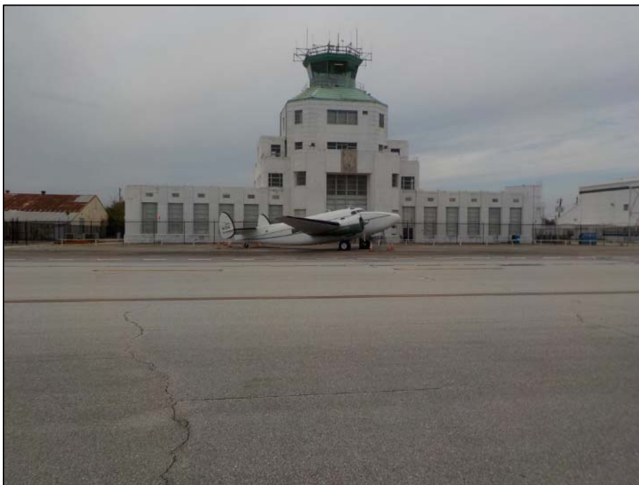
Photo 8. View of the 1940 Air Terminal Museum at the southwestern end of the project limits, facing southwest.
