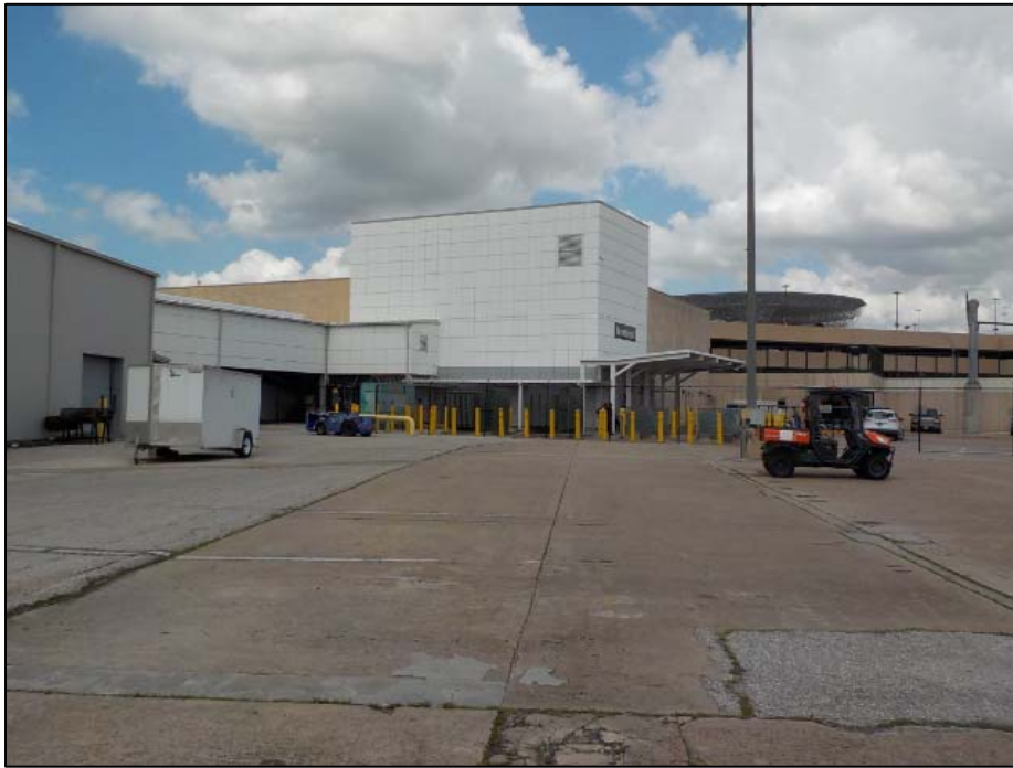
Photo 7. View of the northeast end of the HOU Main Terminal Building, facing southwest.
