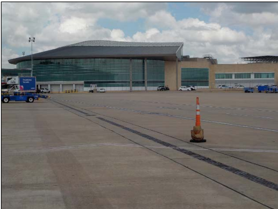
Photo 4. Another view of the eastern side of the HOU Main Terminal Building, facing west.
