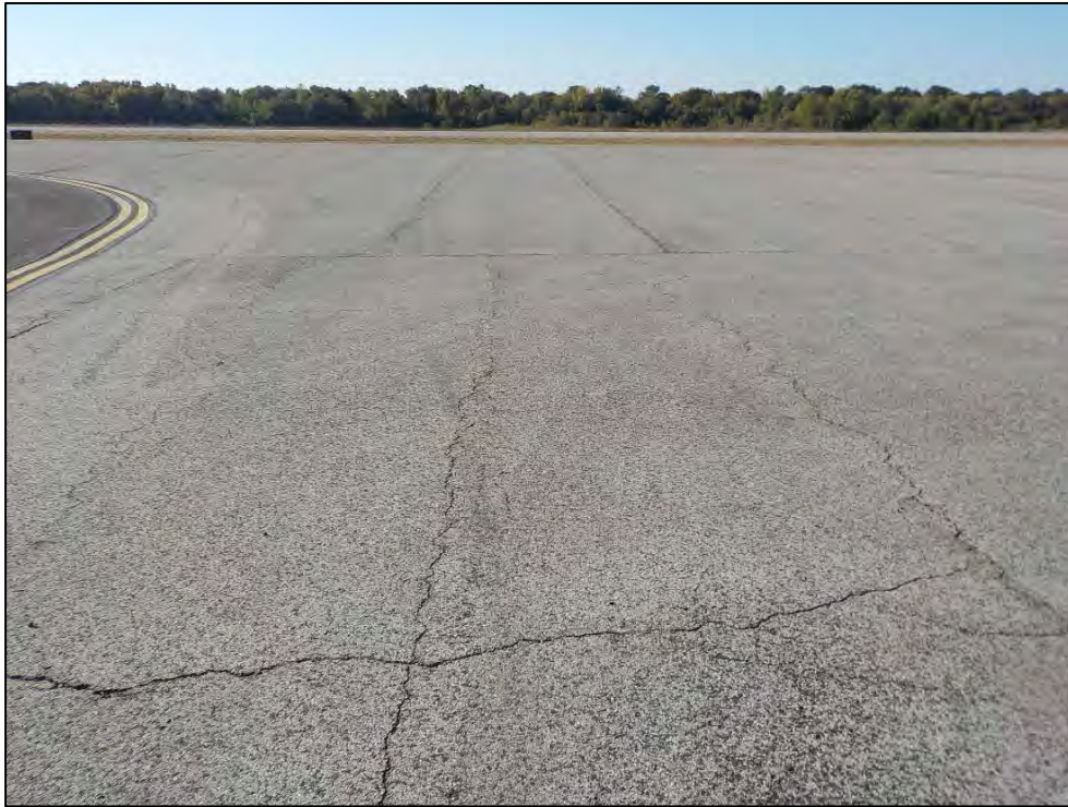
Photo 7. Overview taken near the center of the project area, facing south.
