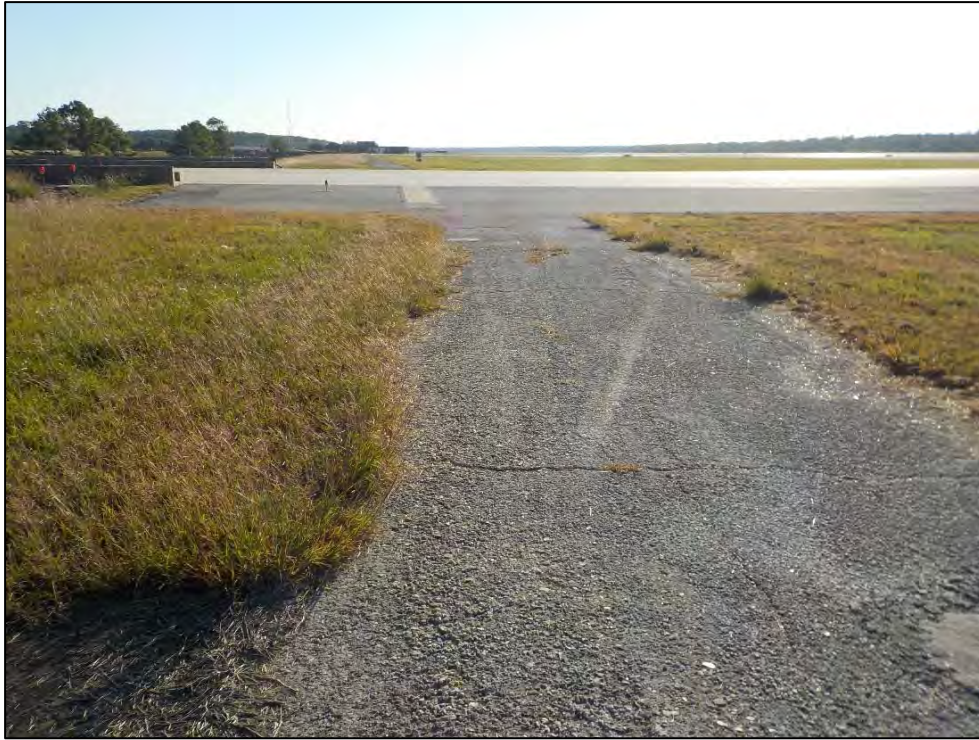
Photo 1. Overview of the project area from the northwest corner, facing east.
