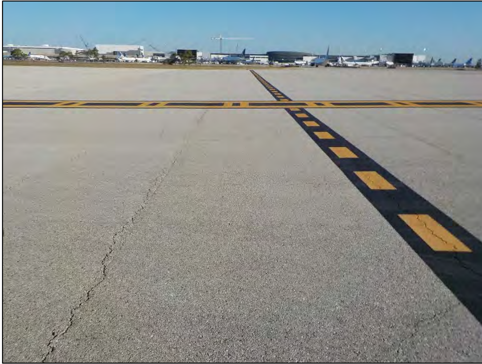
Photo 3. Overview of the project area from the southwest corner, facing north.
