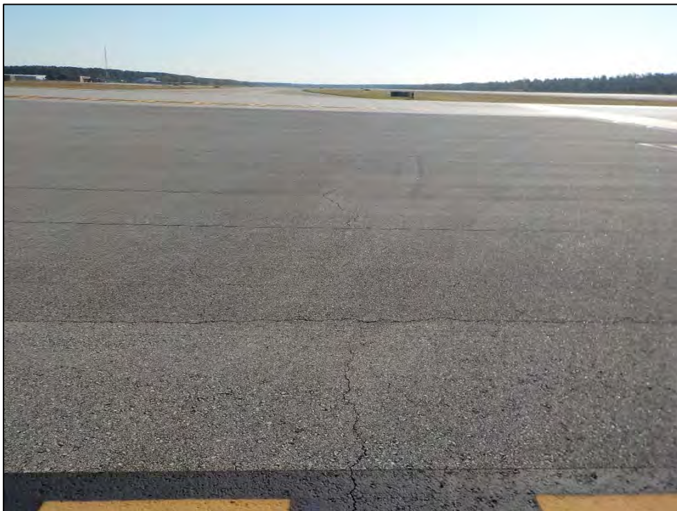
Photo 4. Overview of the project area from the southwest corner, facing east.
