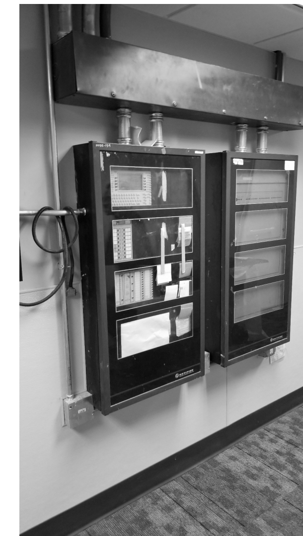
EXISTING FIRE ALARM CONTROL PANEL A
