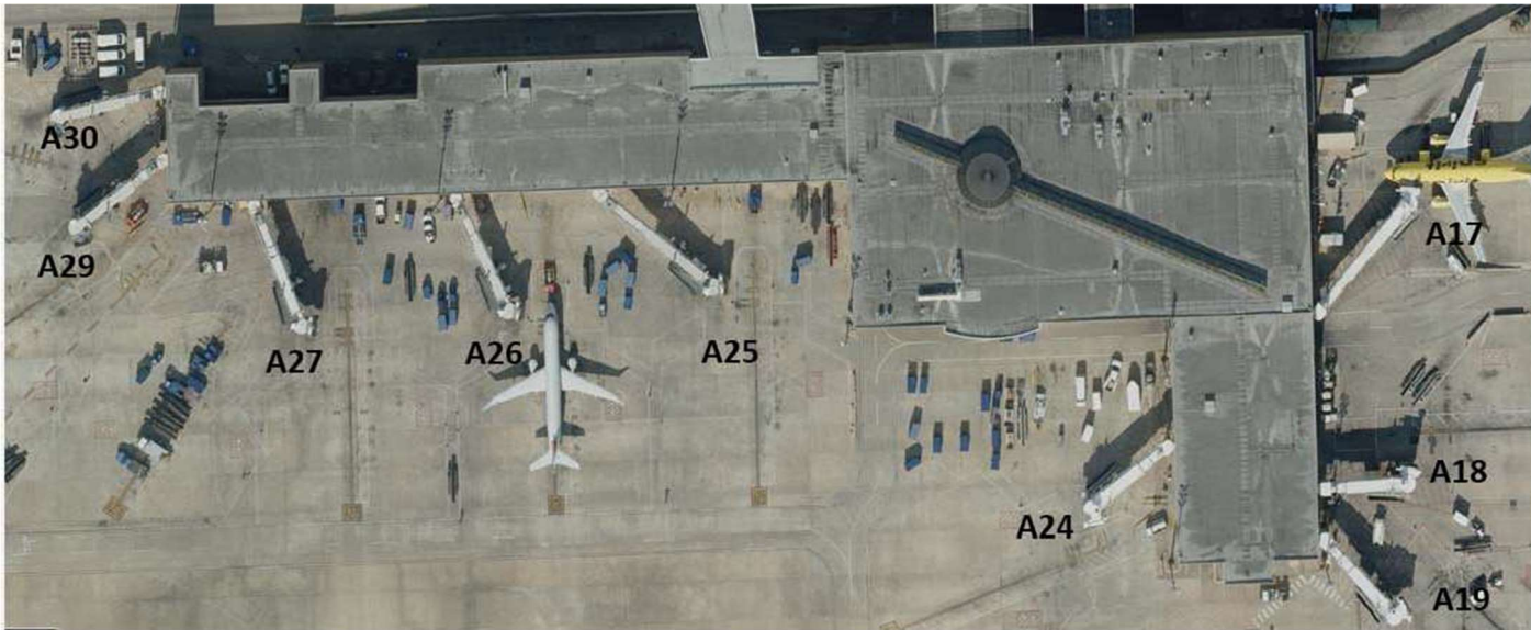
Terminal A South
