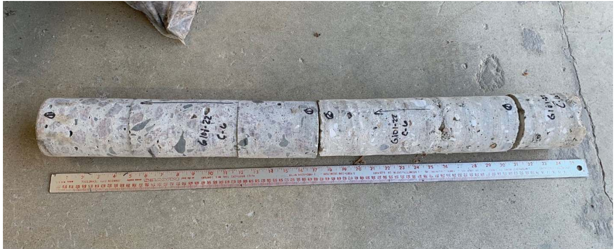
Photo 2 - Core C-6, 16.75" concrete, 16.5 cement-treated base
