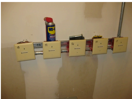
ELEVATOR FIRE RECALL MODULES
