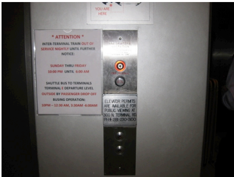
MAIN FLOOR HALL FIXTURE WITH FIRE RECALL SWITCH
