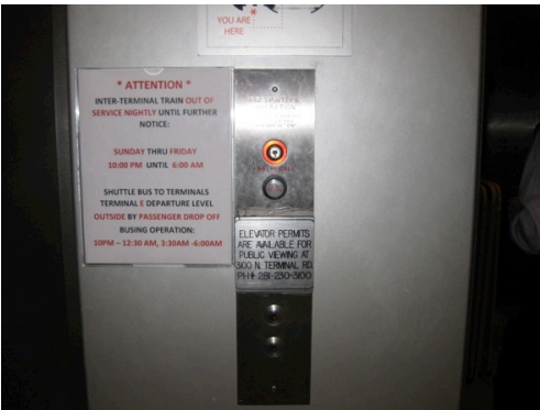
MAIN FLOOR HALL FIXTURE WITH FIRE RECALL SWITCH
