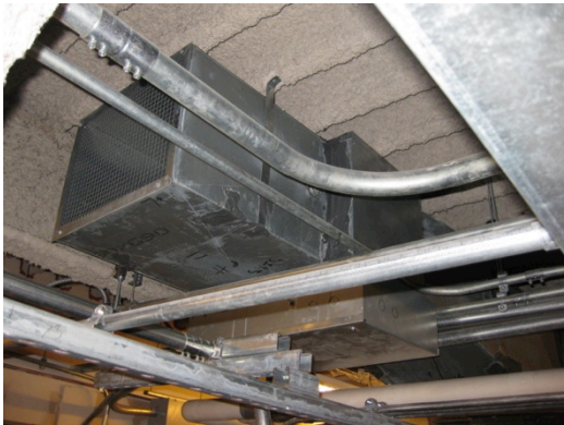
MACHINE ROOM CLIMATE CONTROLL
