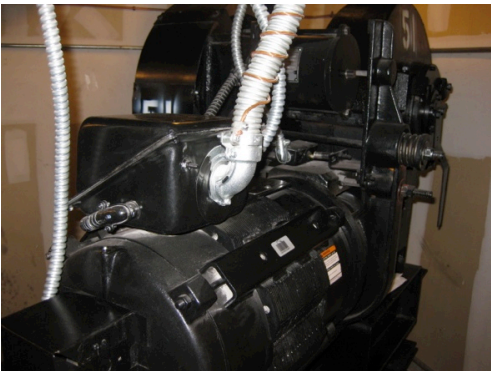
TYPICAL GEARED HOIST MACHINE FRONT VIEW
