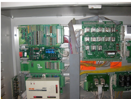
TYPICAL ELEVATOR CONTROLLER
