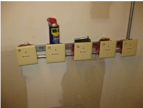
ELEVATOR FIRE RECALL MODULES
