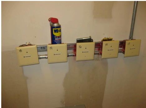
ELEVATOR FIRE RECALL MODULES
