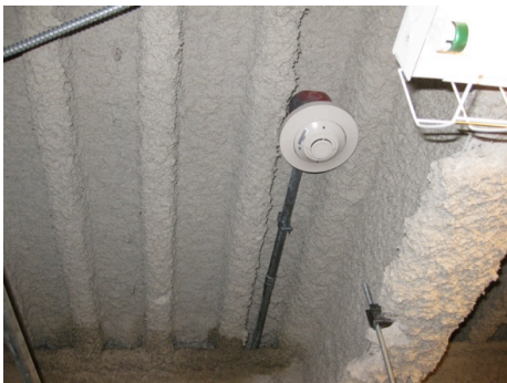
MACHINE ROOM SMOKE DETECTOR
