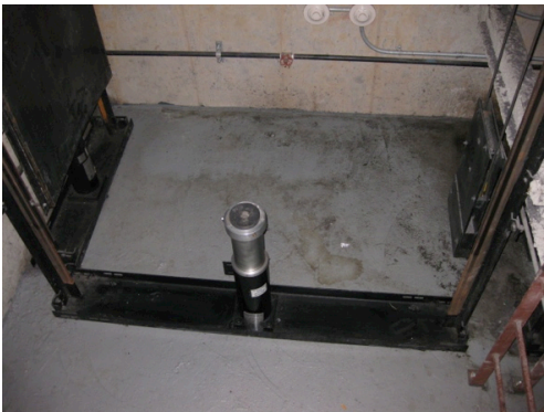
ELEVATOR PIT WITH OIL BUFFER
