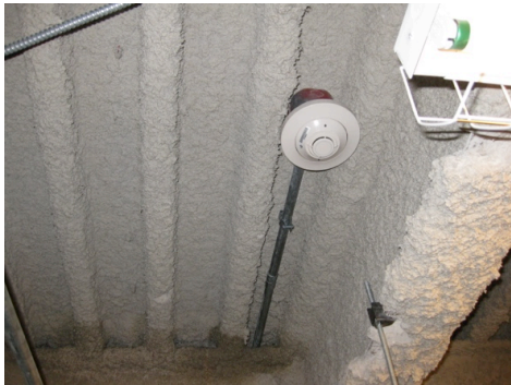
MACHINE ROOM SMOKE DETECTOR
