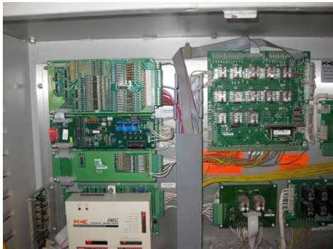
TYPICAL ELEVATOR CONTROLLER
