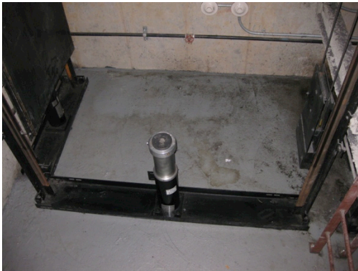
ELEVATOR PIT WITH OIL BUFFER
