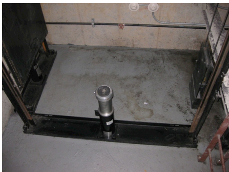
ELEVATOR PIT WITH OIL BUFFER
