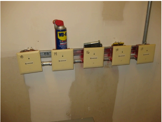
ELEVATOR FIRE RECALL MODULES
