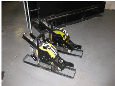
OVERSPEED GOVERNOR ASSEMBLY MOUNTED ON THE MACHINE ROOM FLOOR
