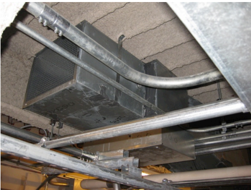
MACHINE ROOM CLIMATE CONTROLL
