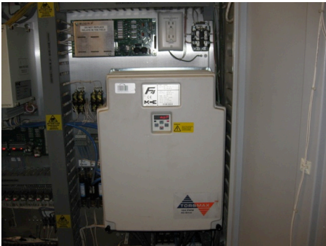
AC DRIVE UNIT MOUNTED IN THE ELEVATOR CONTROLLER
