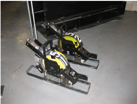
OVERSPEED GOVERNOR ASSEMBLY MOUNTED ON THE MACHINE ROOM FLOOR
