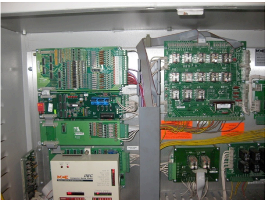
TYPICAL ELEVATOR CONTROLLER
