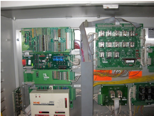
TYPICAL ELEVATOR CONTROLLER
