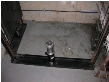
ELEVATOR PIT WITH OIL BUFFER
