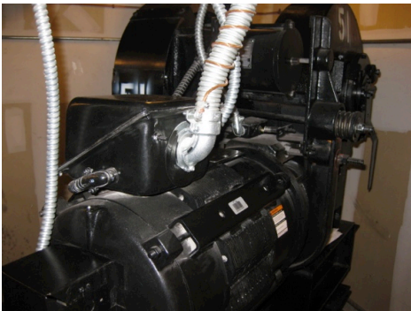
TYPICAL GEARED HOIST MACHINE FRONT VIEW
