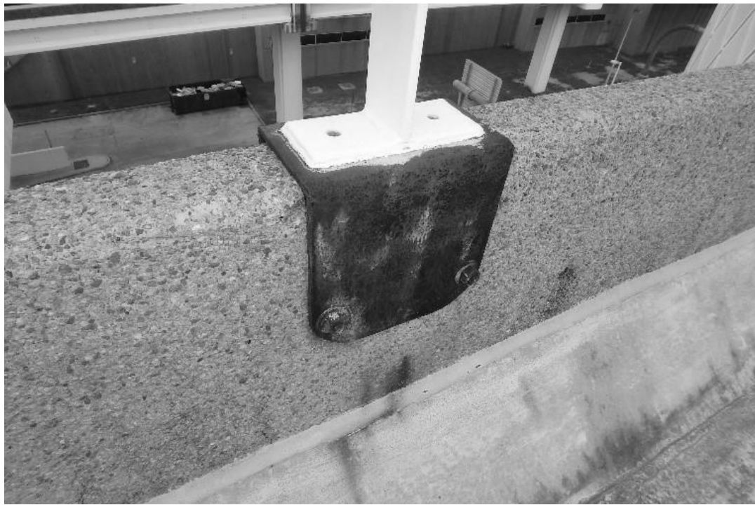
3 CORRODED HANDRAIL CONNECTION NTS
