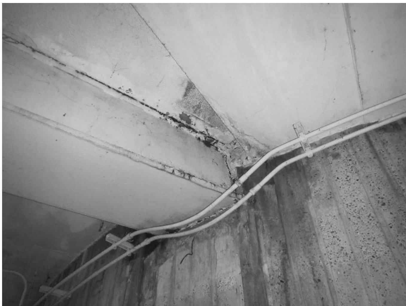
3 CORROSION OF STEEL GIRDER AT WALL CONNECTION NTS
