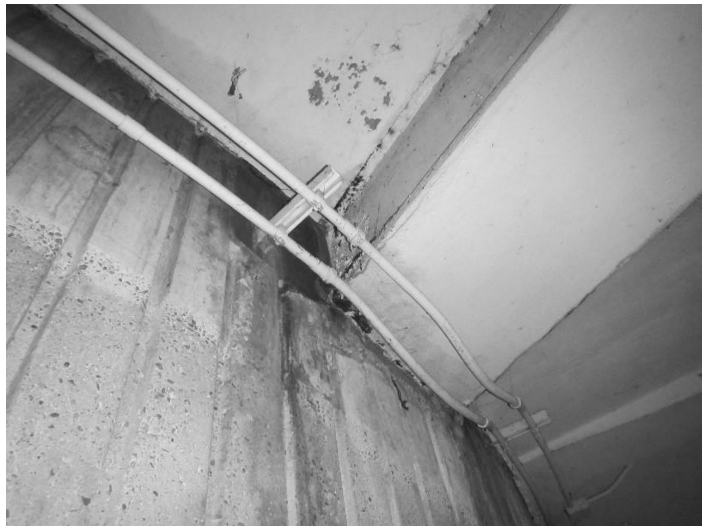
4 CORROSION OF STEEL GIRDER AT WALL CONNECTION NTS
