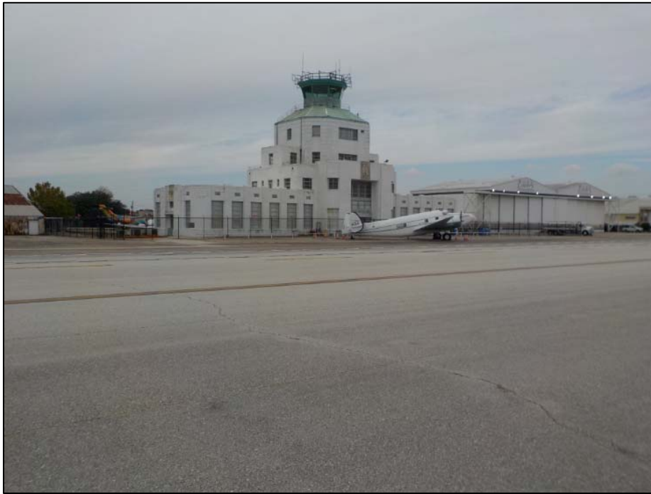
Photo 7. View of the 1940 Air Terminal Museum at the southwestern end of the project limits, facing southwest.
