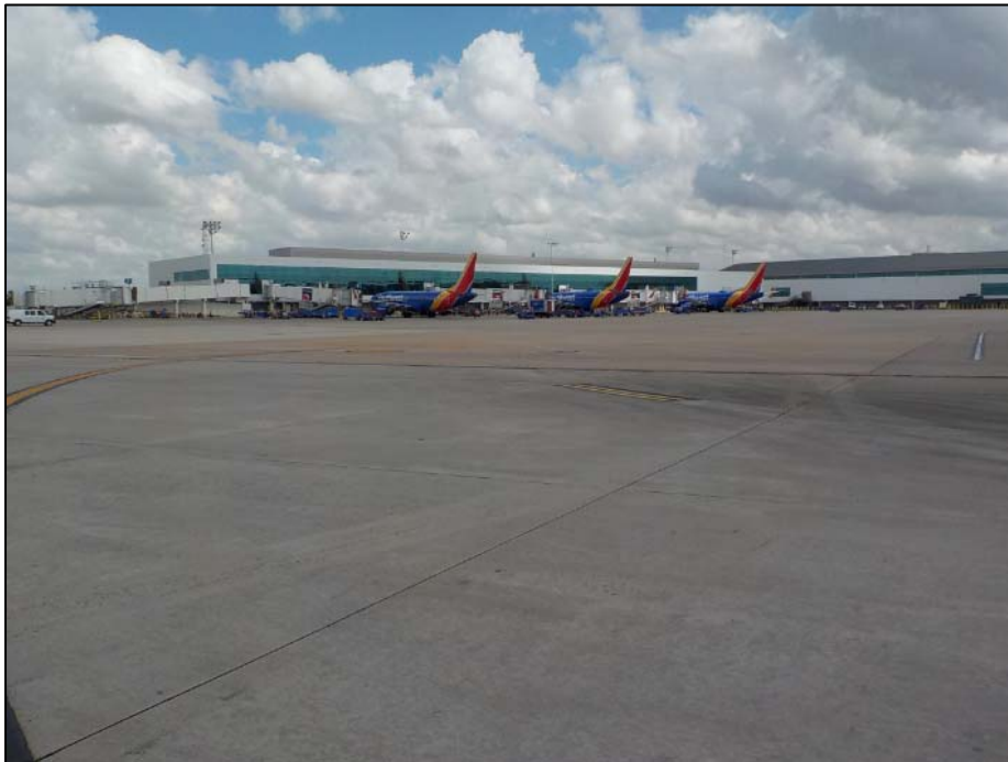
Photo 12. Overview of the West Concourse building, facing northeast.
