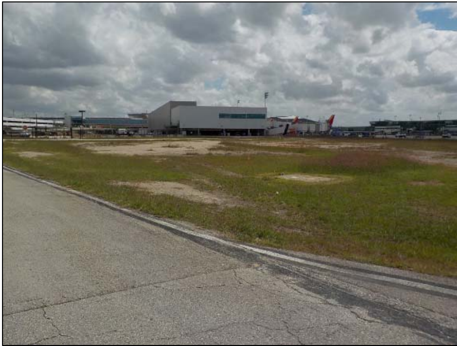
Photo 17. View of the West Concourse Terminal building, facing east.
