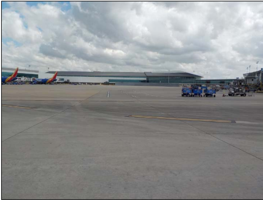
Photo 11. Another overview of the western side of the HOU Central Terminal Building, facing east.
