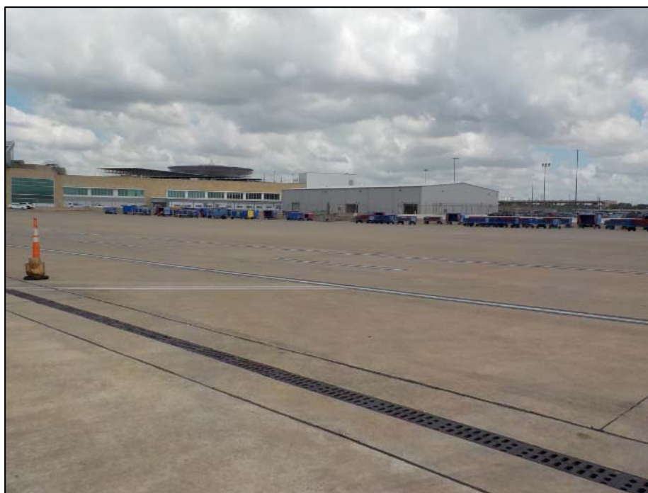
Photo 6. View of the northeast end of the HOU Main Terminal Building and taxiway, facing northwest.
