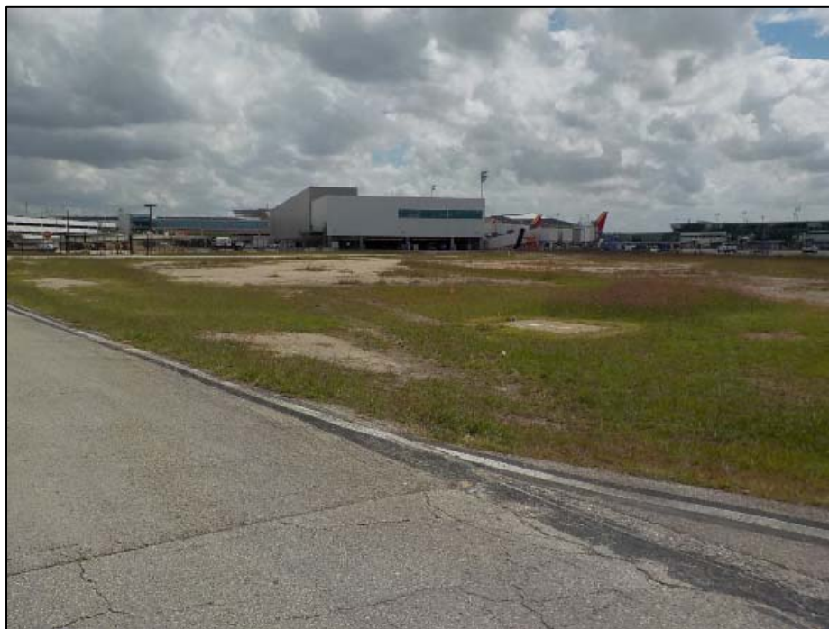
Photo 17. View of the West Concourse building, facing east.
