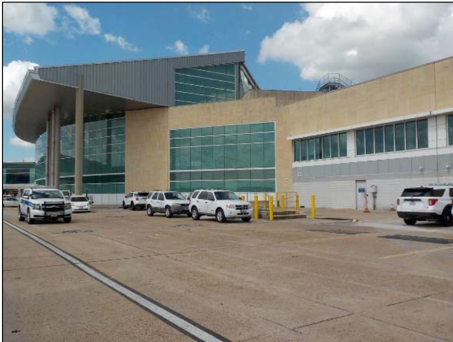
Photo 8. View of the eastern side of the HOU Central Terminal Building, facing southwest.
