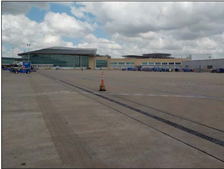
Photo 3. Overview of the eastern side of the HOU Main Terminal Building, facing west.
