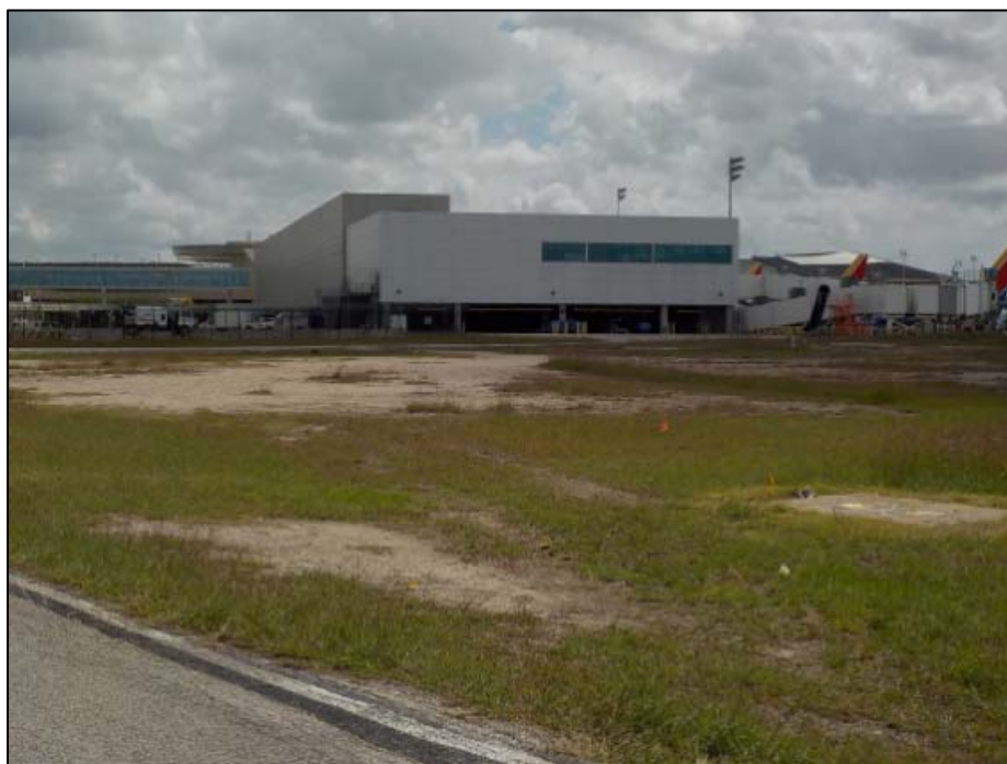
Photo 18. Another view of the West Concourse building, facing east.
