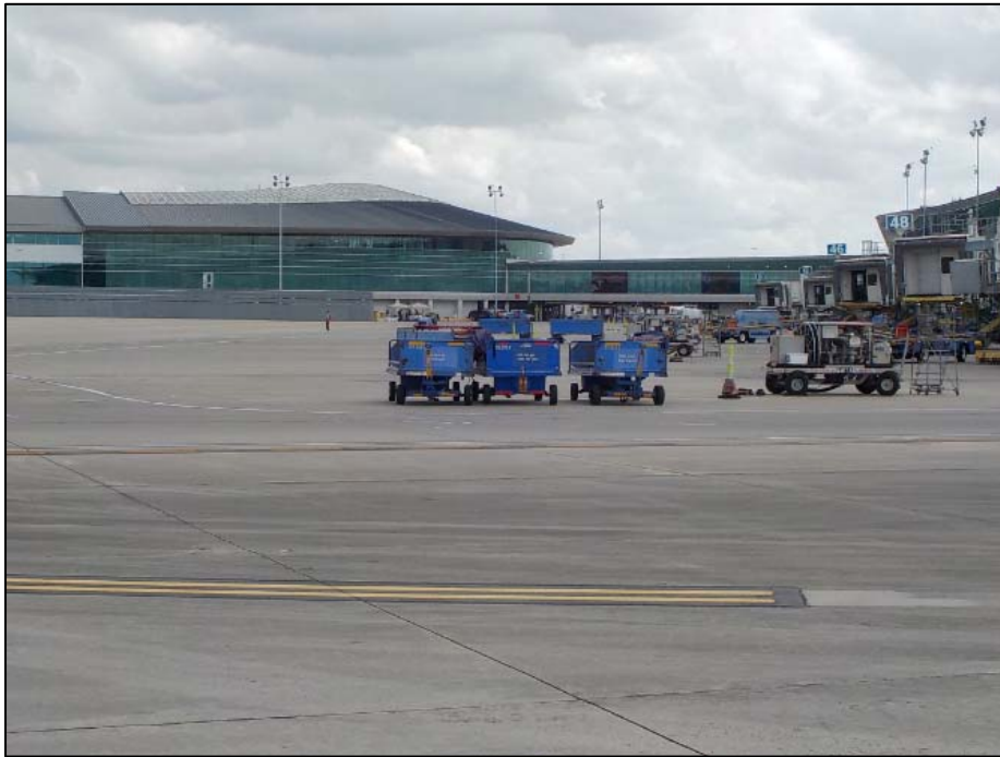
Photo 9. View of the western side of the HOU Main Terminal Building, facing east.
