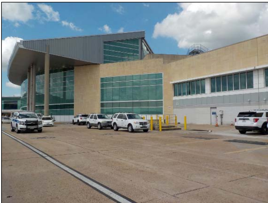
Photo 8. View of the eastern side of the HOU Main Terminal Building, facing southwest.
