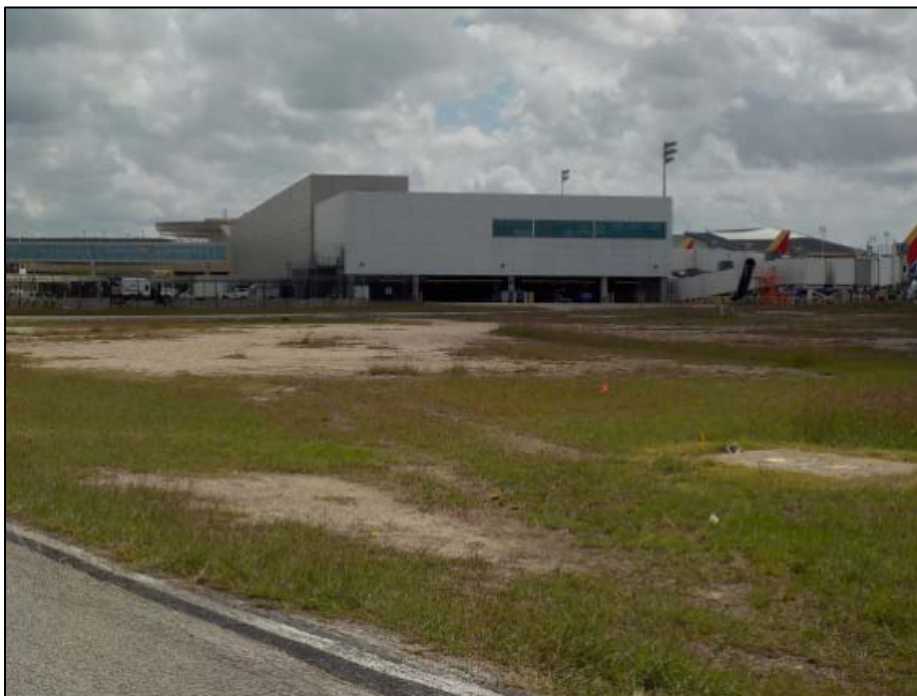
Photo 18. Another view of the West Concourse Terminal building, facing east.
