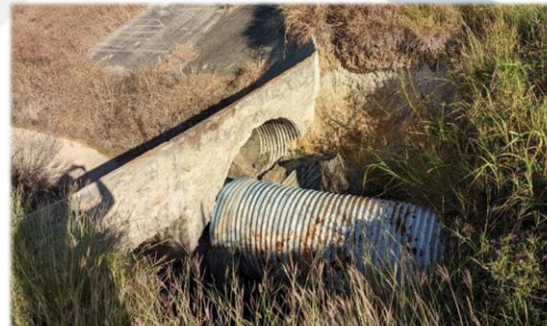
Figure 4 – North Culvert Headwall Erosion
