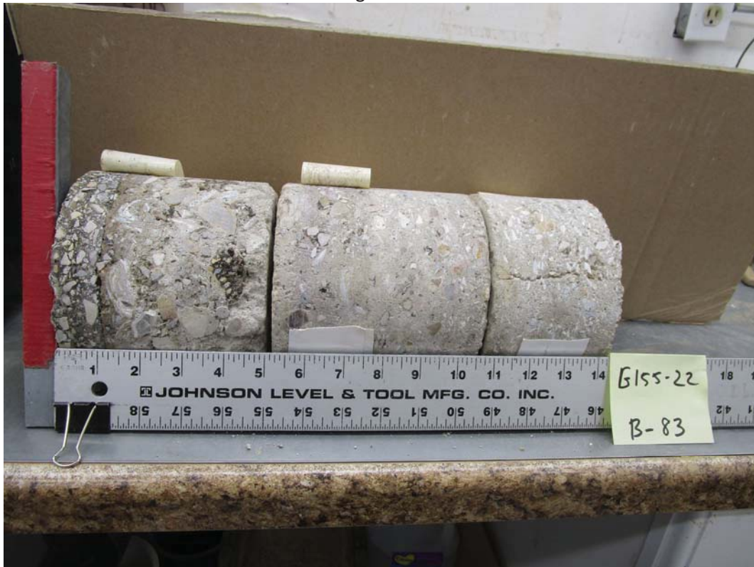
Photo 02 - Boring B-83 Pavement Core
