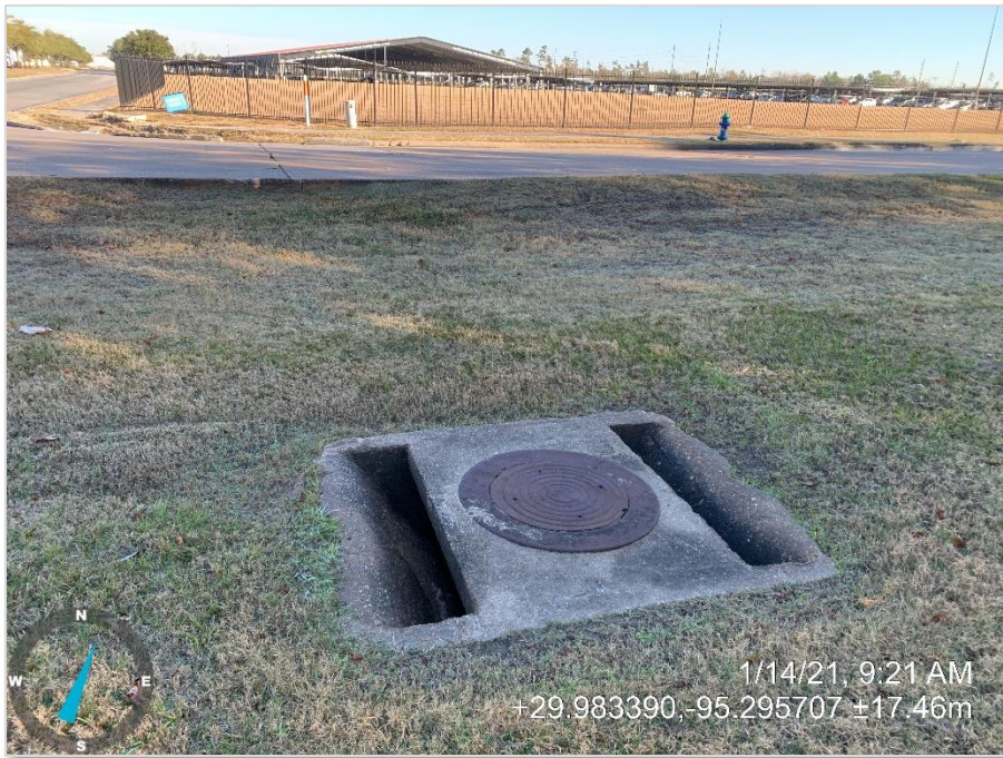
4. Typical representation of the drains in the maintained grass along both sides of the median adjacent to Will Clayton Parkway.
