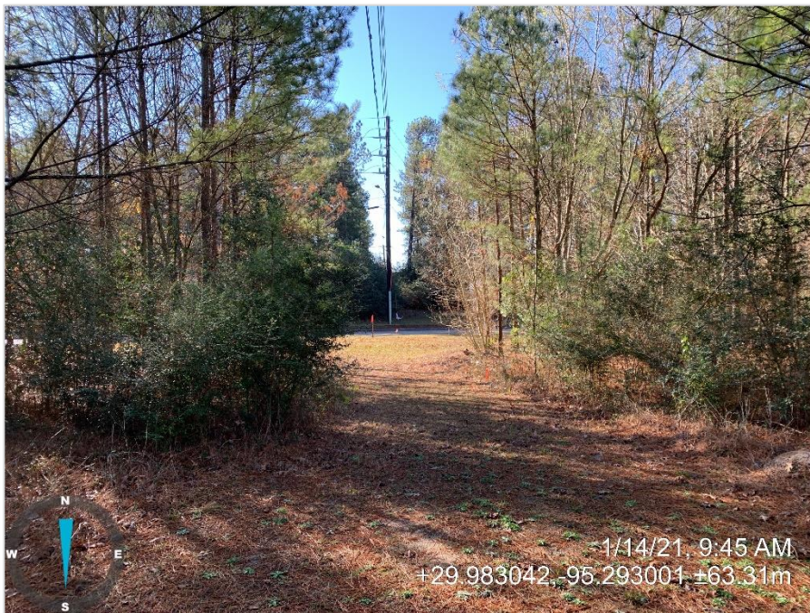
4. Facing south. Transmission lines observed transecting the median area of Will Clayton Boulevard.
