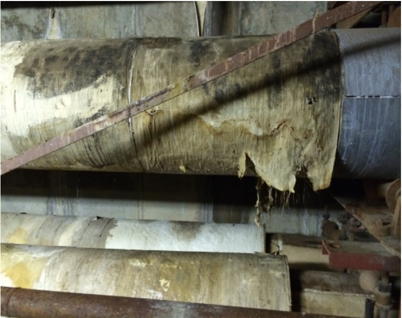
Figure 8-6 Deteriorating Insulation in Tunnel
