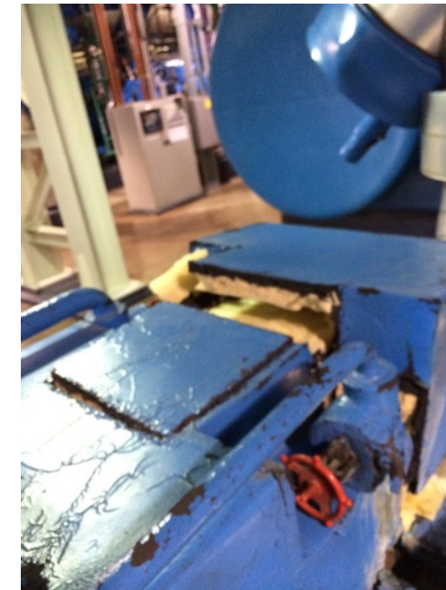
Figure 8-2 Cracked Insulation on CHP-10
