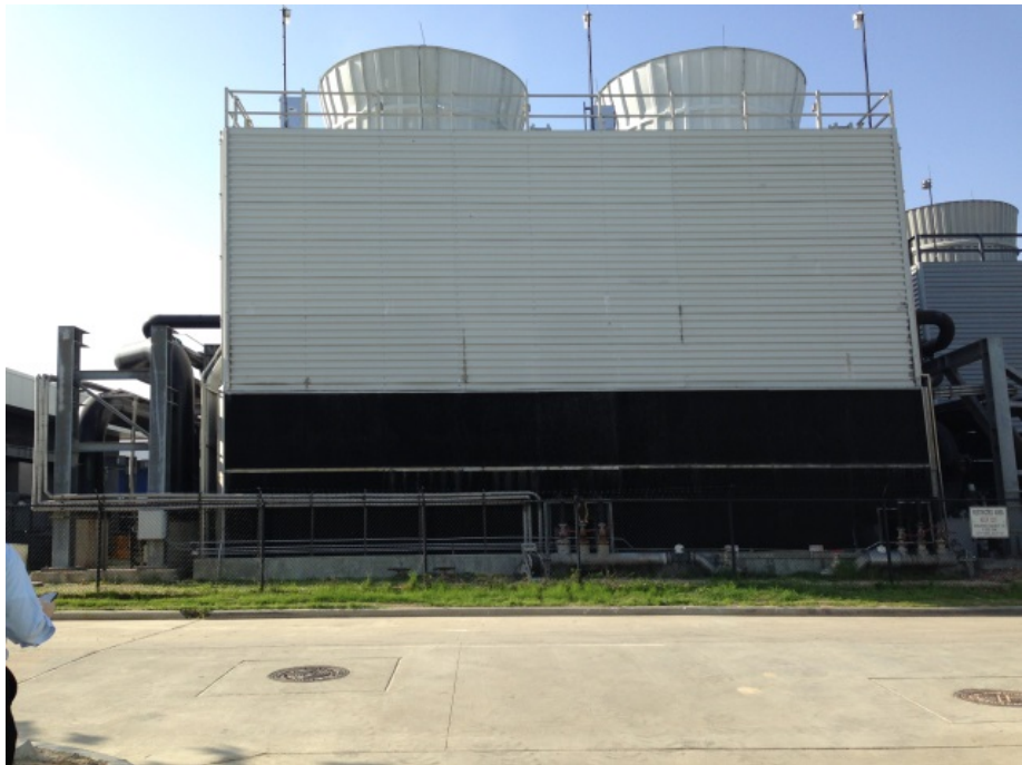
Figure 8-3 Wrong Fill in Cooling Towers
