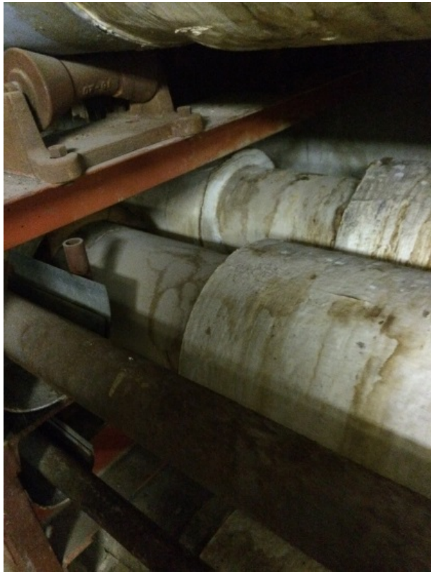
Figure 8-5 Missing Insulation in Tunnel Piping
