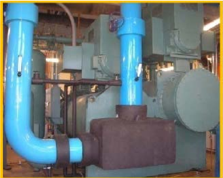
Figure 5-1 Heat Pump Chiller
