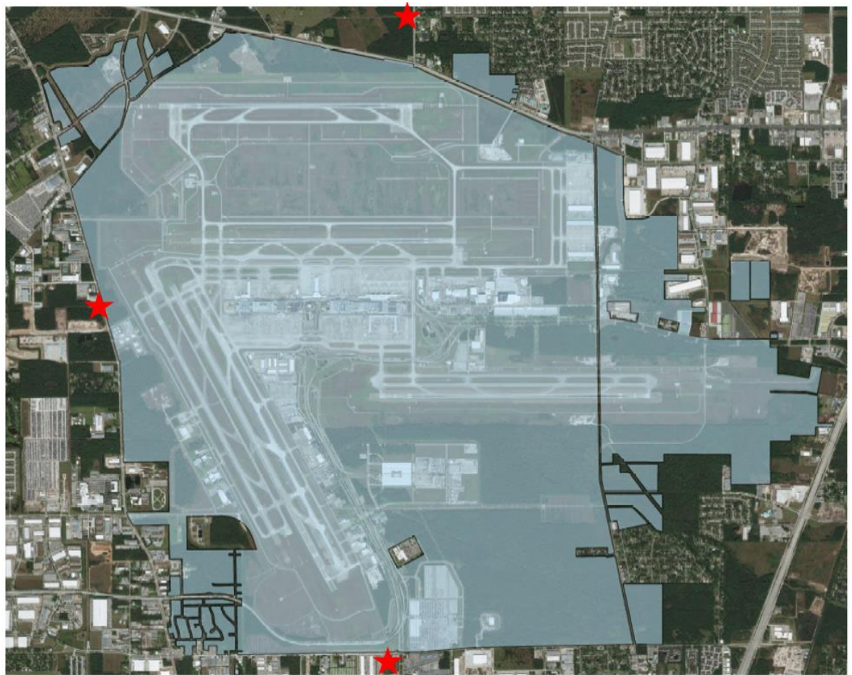
Figure 1 IAH Property and Available green space for solar and other Energy Resource Measures
