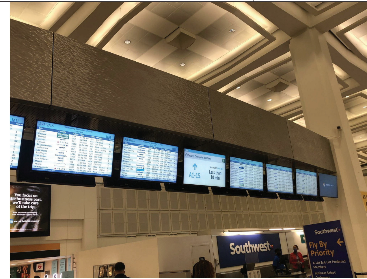
AREA 2 - PHOTO OF EXISTING CONDITION
