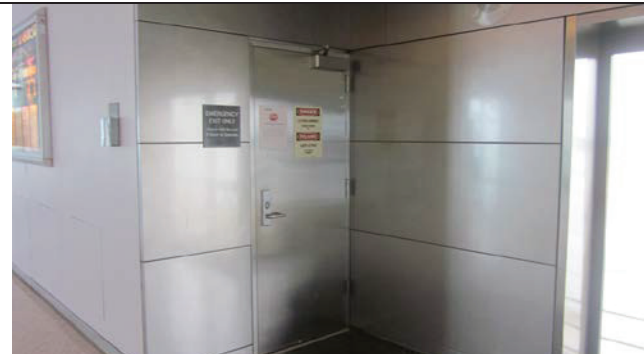
General view of wall panel
