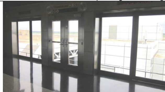
Typical entry area to APM, panel on ceiling and walls
