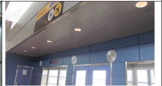
Typical entry area to APM, panel on ceiling and walls
