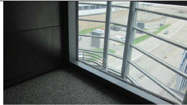
General view of windows with paneling and caulking
