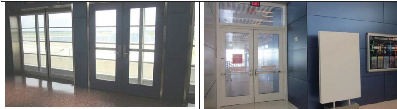
Typical entry area to APM, panel on ceiling and walls
