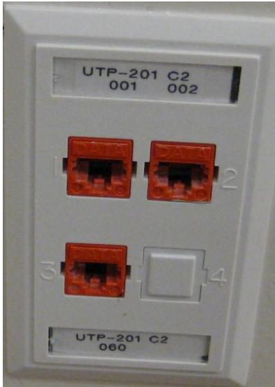
Outlet label placement 4-port: under top-aligned, Plexiglas cover – servicing IDF identifier over port identifiers. Ports should be identified left-to-right. Under bottom-aligned, Plexiglas cover – servicing IDF identifier over port identifiers. Ports should be identified left-to-right. Follow 3-port example.
