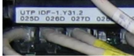
Regarding switches: generally space does not allow for switch port labeling; ports must be identified however in order to correlate circuit connectivity to/from/through the device.
