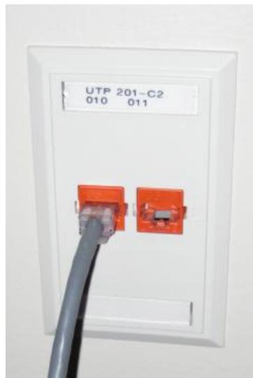
Outlet label placement 3-port: under top-aligned, Plexiglas cover – servicing IDF identifier over port identifiers. Ports should be identified left-to-right. Under bottom-aligned, Plexiglas cover – servicing IDF identifier over port identifiers. Ports should be identified left-to-right.
