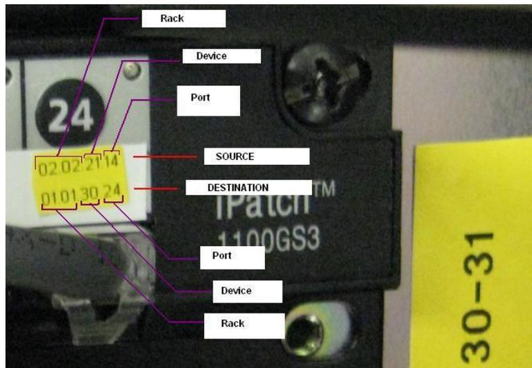
All port identifiers follow some specific schema; new ports must be identified accordingly. In the event that a determination cannot be made regarding the identity of the port, please contact the iPatch database administrator prior to documenting.
