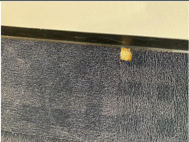
Terminal C Carpet with Mastic
