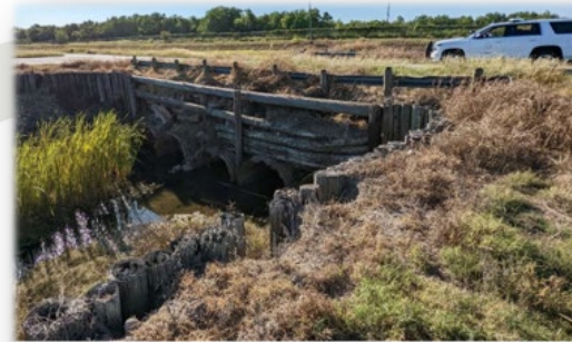
Figure 2 – Ditch C Existing Outfall
