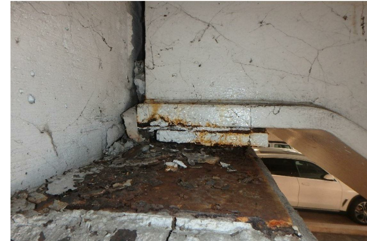
5 CORRODED STEEL PLATES IN SLIDE BEARING ASSEMBLY - LEVEL 5 NO SCALE WPM 19
