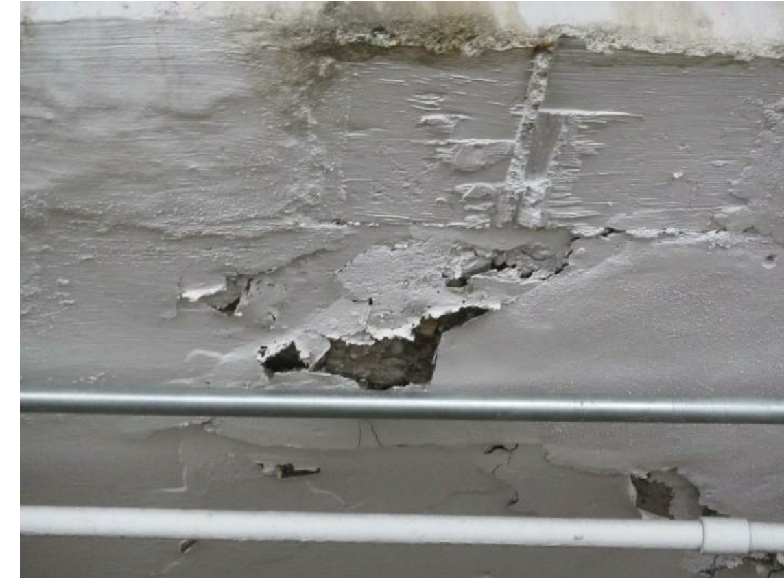
1 SPALLED CONCRETE AT UNDERSIDE OF BRIDGE - LEVEL 6 NO SCALE WPM 02
