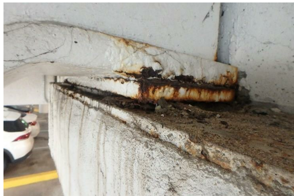
4 CORRODED STEEL PLATES IN SLIDE BEARING ASSEMBLY - LEVEL 6 NO SCALE WPM 09
