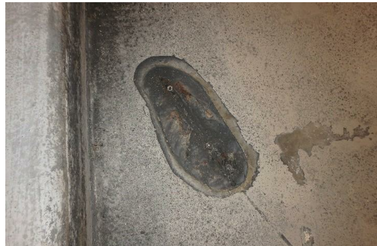
2 SPALLED CONCRETE IN TOPPING SLAB - TYPICAL CONDITION NO SCALE WPM 29
