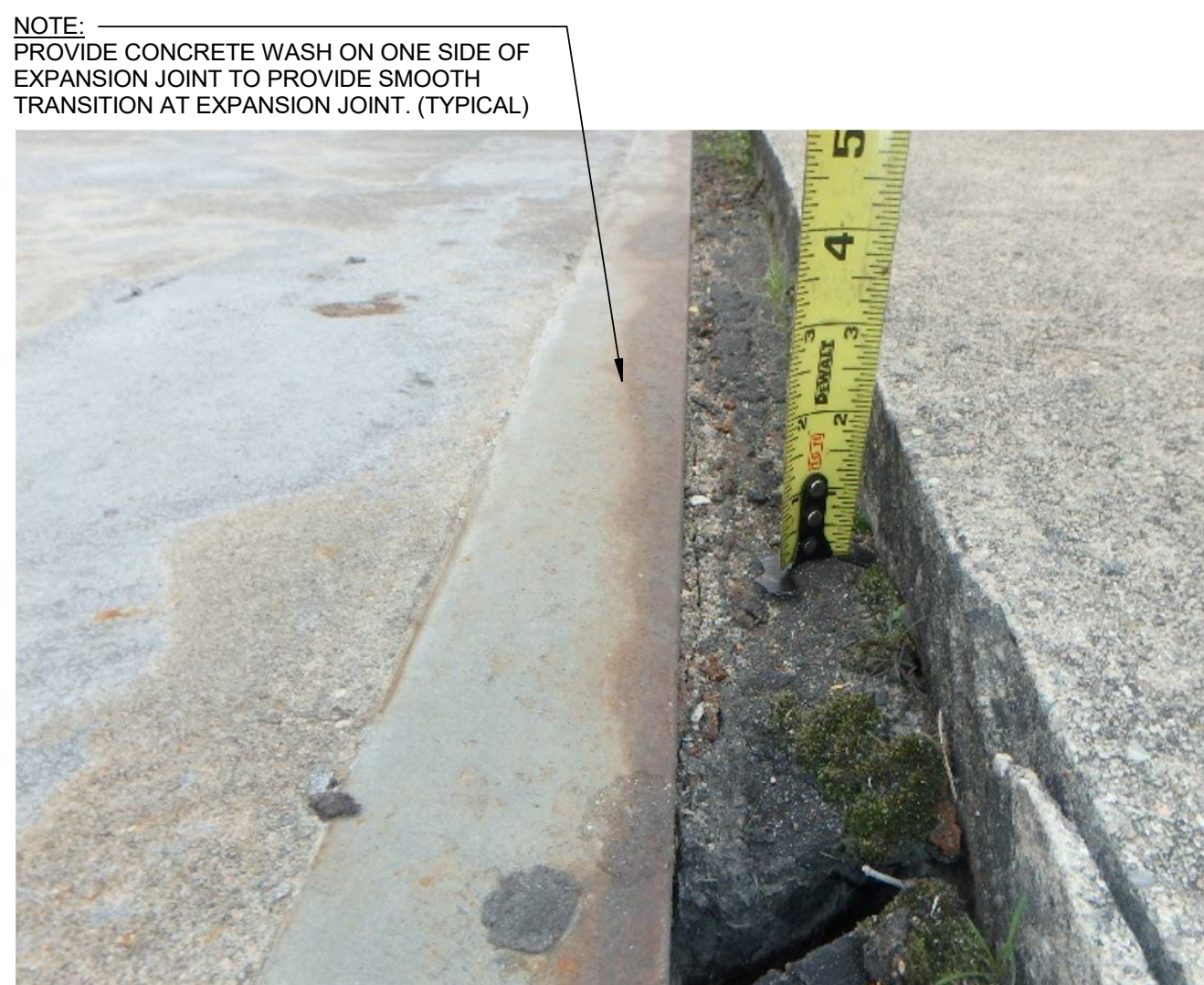
11 EXPANSION JOINT FAILURE AND VERTICAL SEPARATION IN SLAB NO SCALE WPM 34
