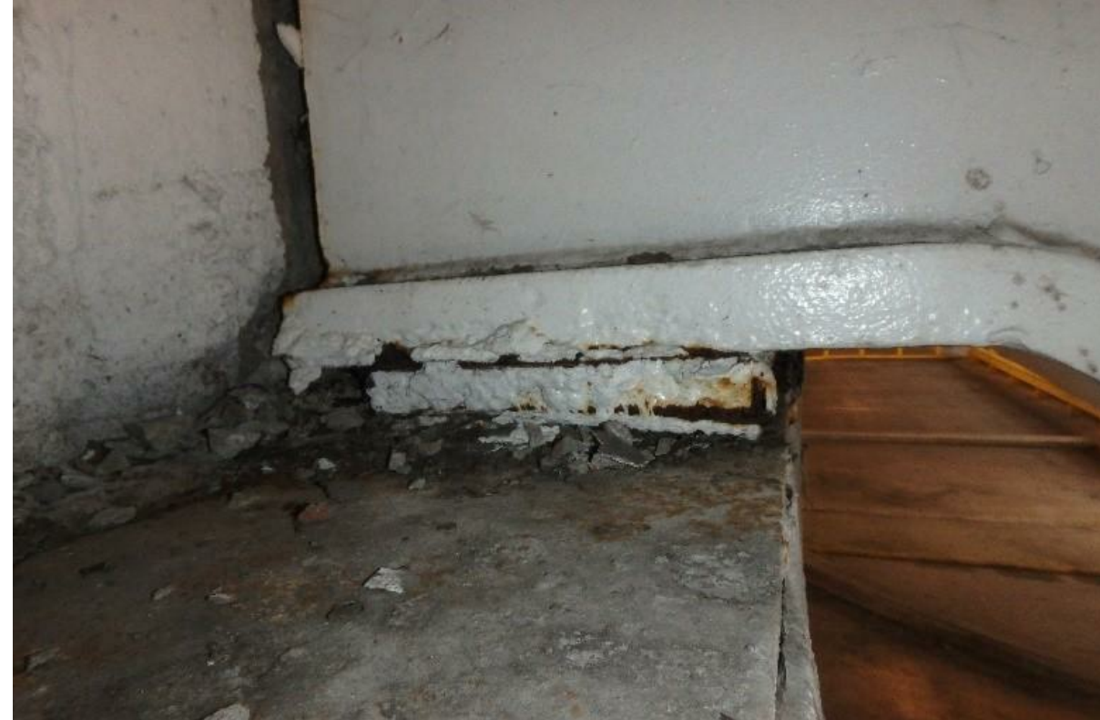
3 CORRODED STEEL PLATES IN SLIDE BEARING ASSEMBLY - LEVEL 5 6" = 1'-0" WPM 15
