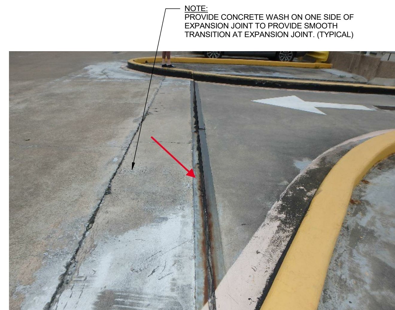
10 EXPANSION JOINT DETERIORATION - TYPICAL CONDITION NO SCALE WPM 33
