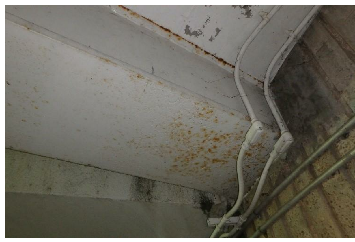
7 CORROSION OF STEEL BOX GIRDER - TYPICAL CONDITION NO SCALE WPM 23
