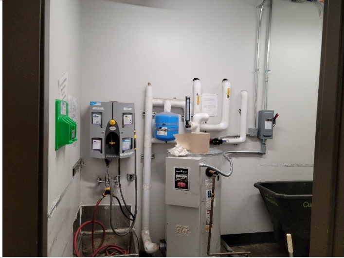
Photo 9: Interior view of JC1.
