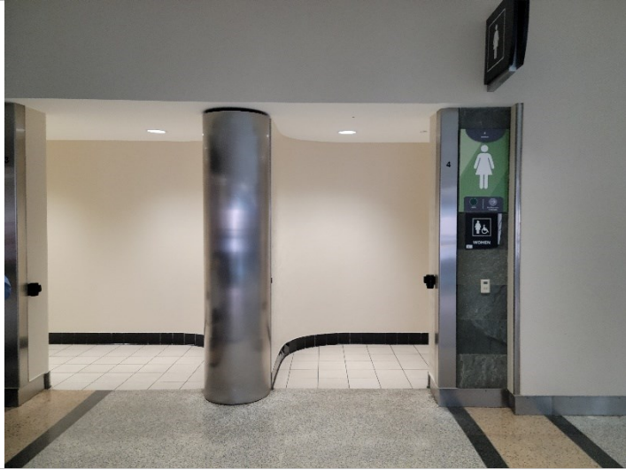
Photo 1: View of area of Restrooms 3, 3A, 4, and JC3.
