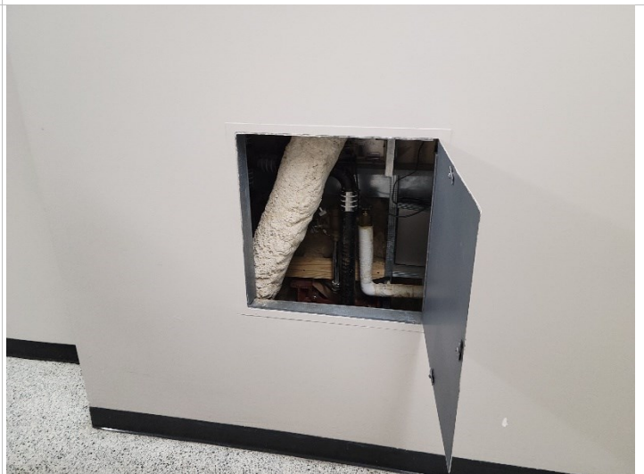
Photo 4: View of cabinet adjacent to Restroom 3A.
