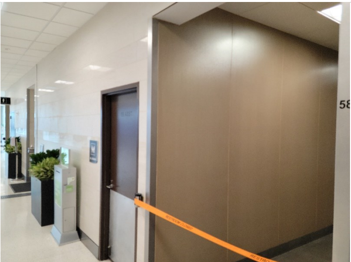
Photo 8: View of area of Restrooms 58, 58A, 59, and JC1.
