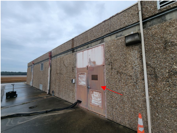
Building Exterior – Sample 1 (Red Door)
