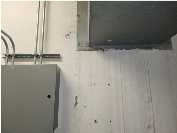
HA 1: Textured/Painted White Concrete Wall
