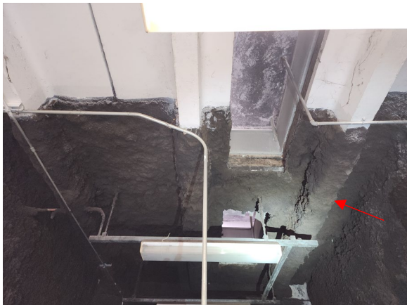
HA 6: Black Fireproofing Insulation on Concrete
