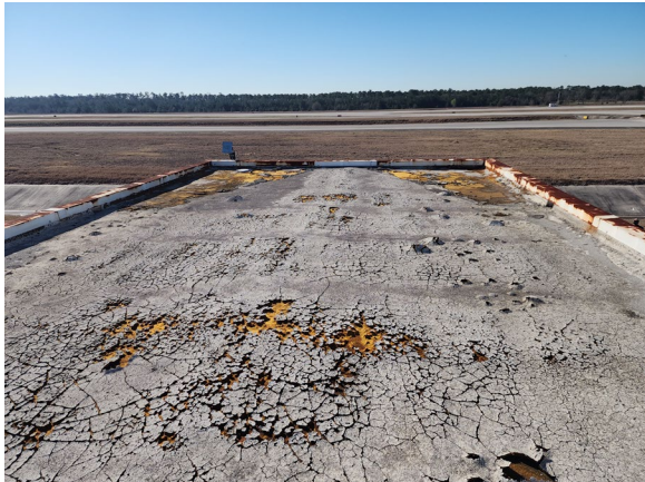
HA 2: Polyurethane Foam Roof
